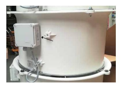
The sticker on the side of the electrical box indicates the type of power supply for which the motor has been configured. For connection to the main line, refer to the USE and MAINTENANCE manual
